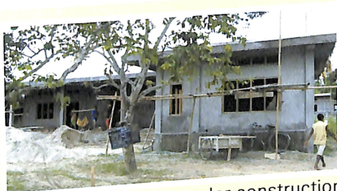
Lab cum class room under construction
